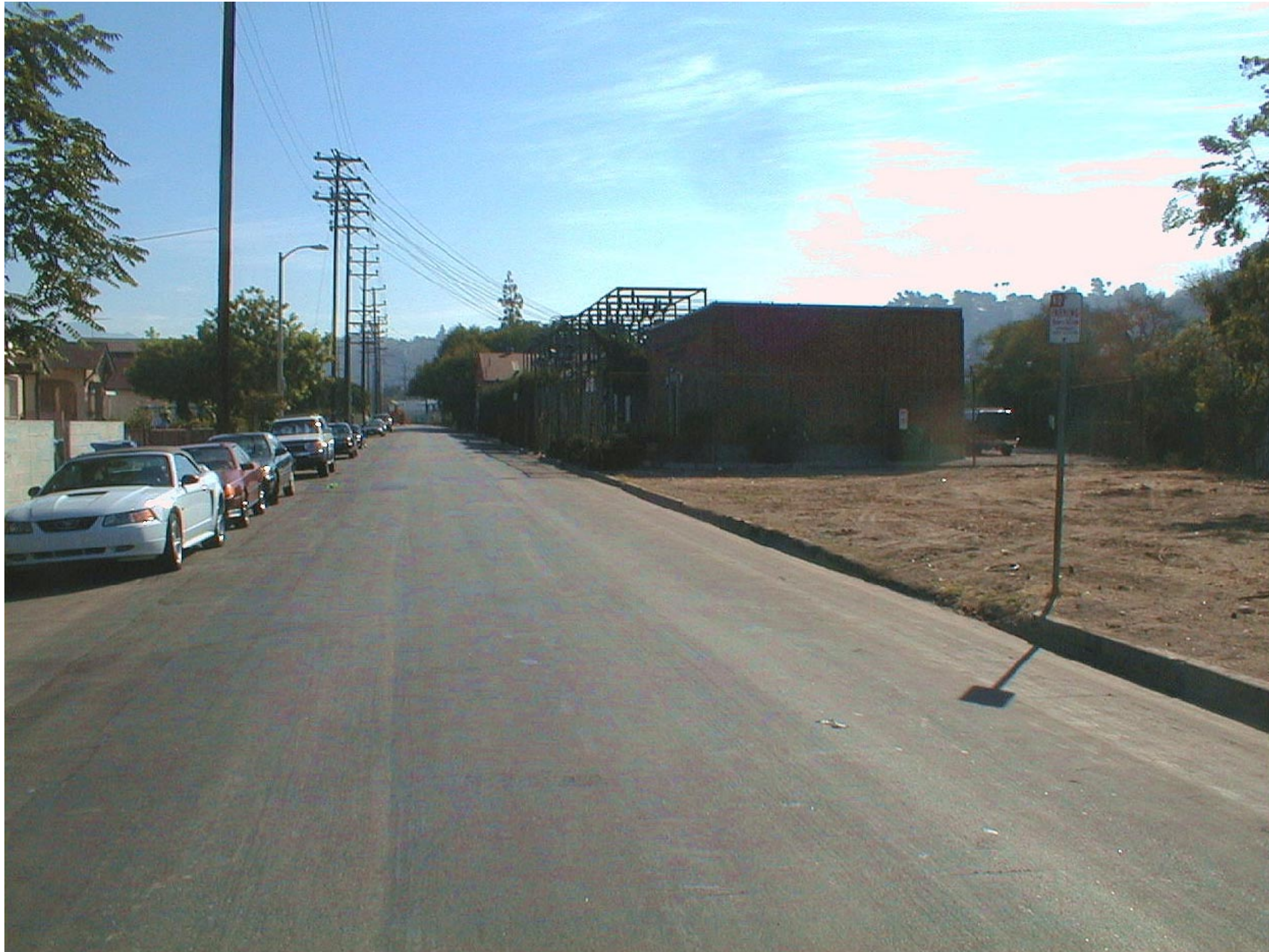
MARMION WAY LOOKING NORTH TOWARD FRENCH AVE STATION
